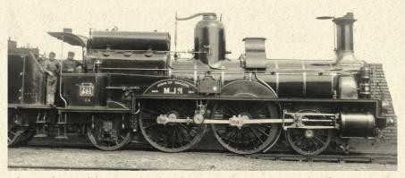
This relatively rare 1'B1' axle arrangement was built more frequently in 1875. The rear trailing axle actually made it possible to carry a larger boiler without compromising stability. On tender locomotives, the rear trailing axle carried the weight of the water tanks, the coal bunker, and the cab. Locomotives of this type are located primarily in Great Britain, Belgium, and France. The PLM locomotive shown here was rebuilt in 1922 as 0-8-0T locomotive No. 7702.
